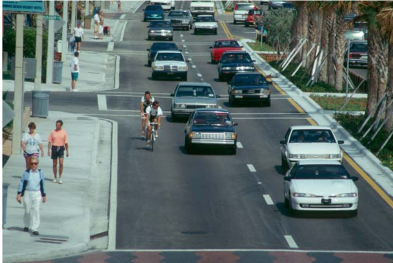
An example of a wide outside lane bike facility & an attached sidewalk This should be done mainly on low speed low volume roads.
