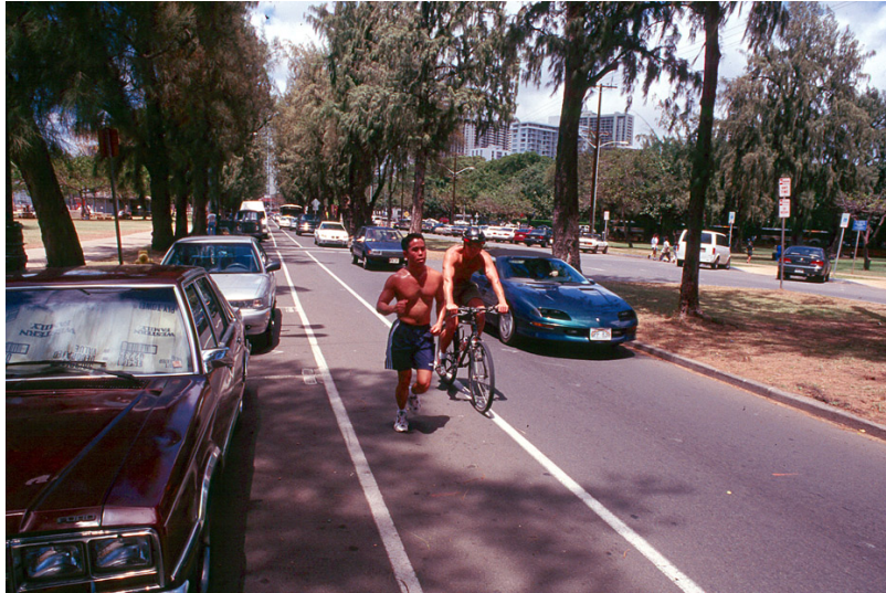
Boulevard with Parking Lane, Bike Lane, Raised Median This example provides a relatively safe area for all users of the roadway.
