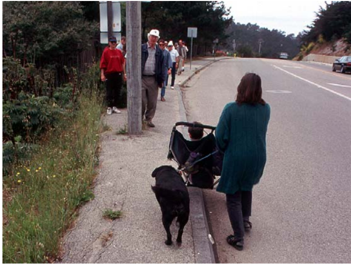
A poor example of an attached sidewalk with utility features in the way Note how the utility pole forces some pedestrians onto the road.
