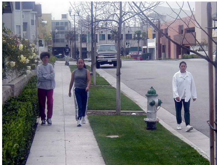
Detached sidewalk with trees in the buffer strip Note location of fire hydrant which is out of the pedestrian's way.
