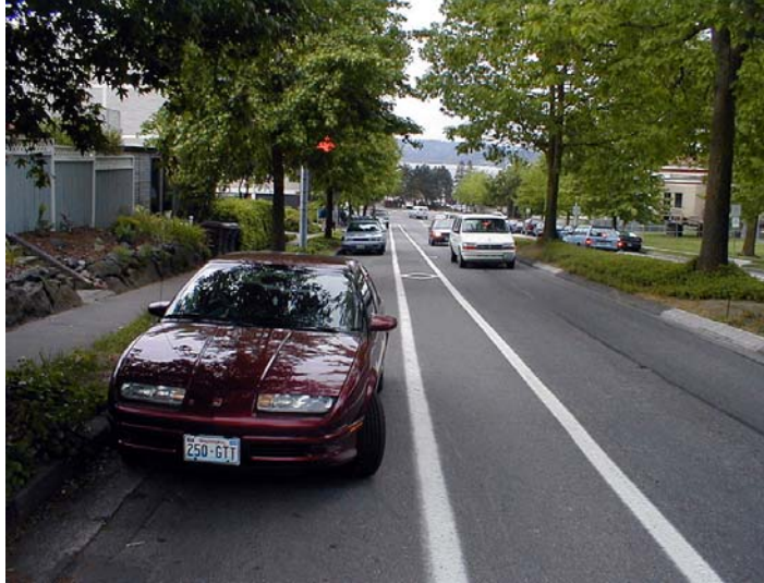
Boulevard with detached sidewalks, bike lanes, and raised planted median This provides a very secure area for pedestrians and bicyclists and helps to slow traffic.
